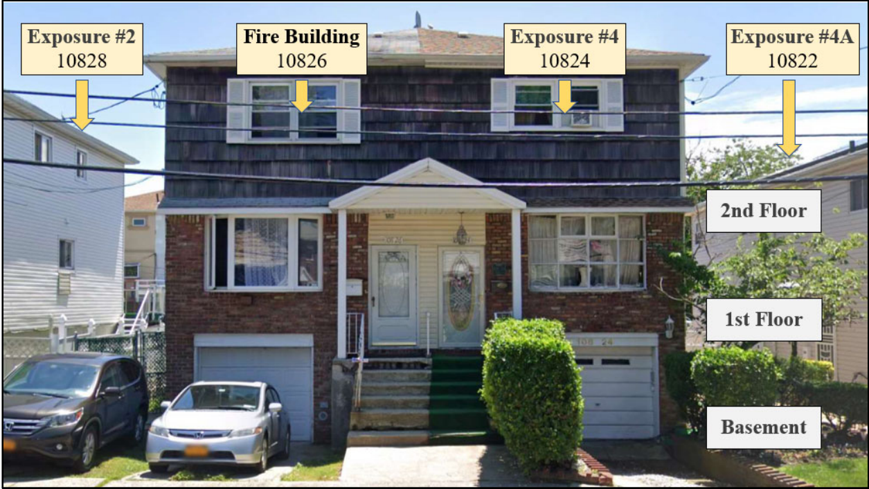
Figure 1. Building and floor designations during the incident.
