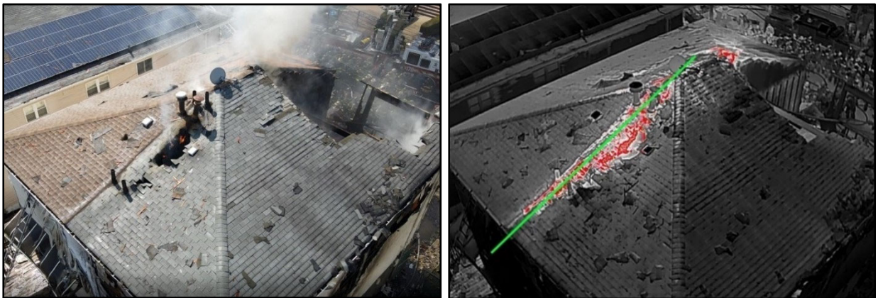
Figure 43. Photos of the top rear section of the Fire Building and Exposure #4 Building with thermal imaging, courtesy of FDNY Robotic Unit Drone. The green line represents the top of the demising wall showing heat and fire on both sides.
