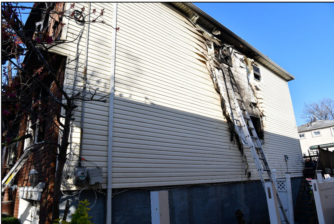
Figure 29. Placement of the L103 OV Firefighter's 24-foot portable ladder against the second-floor window on the exposure #4 side of 10824 Avenue N.
