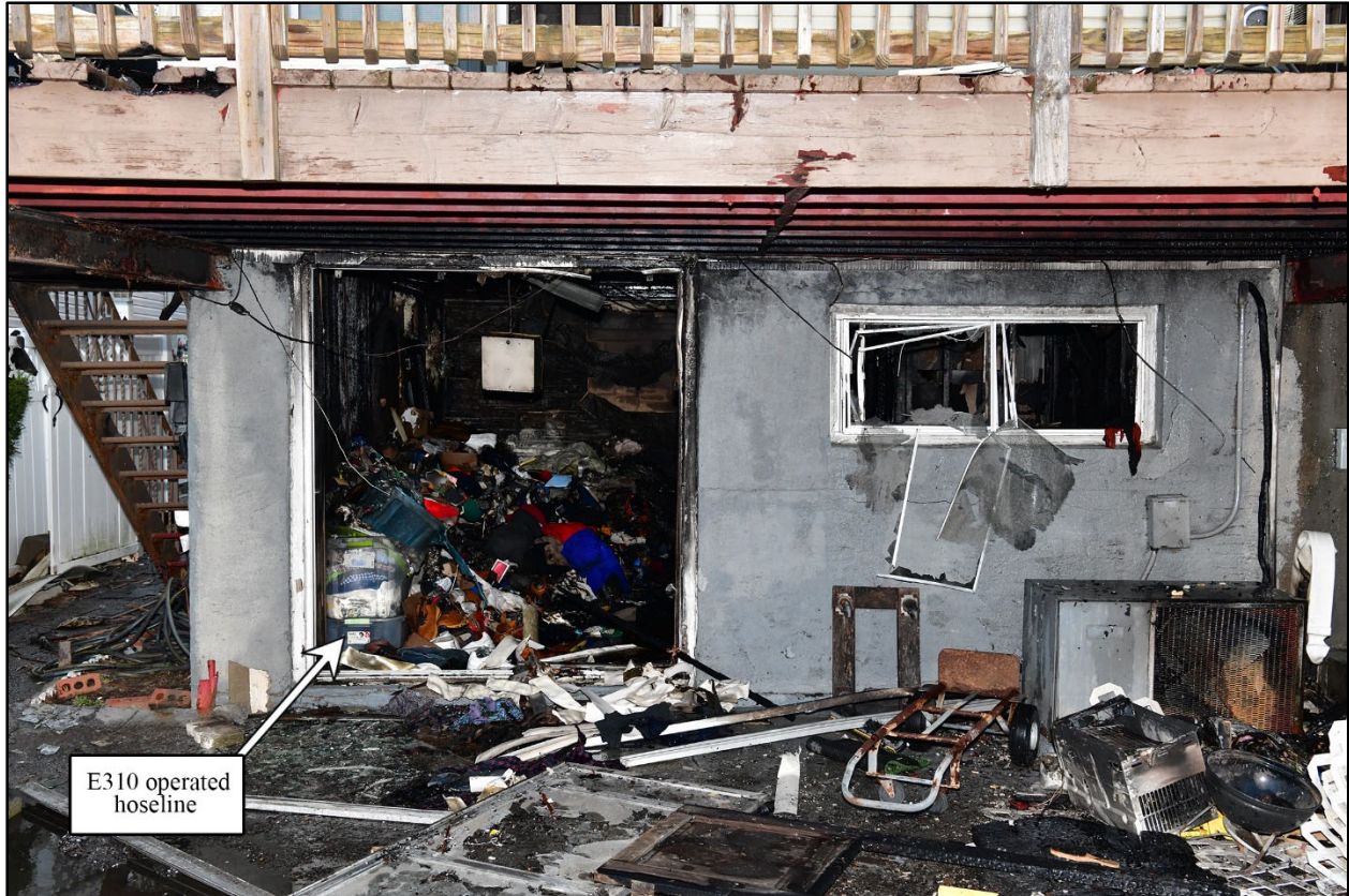
Figure 38. View of the rear basement level of 10824 Avenue N.
