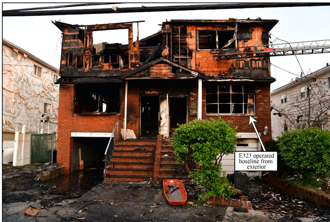
Figure 37. E323's hoseline placement and operation at 10826 and 10824 Avenue N.
